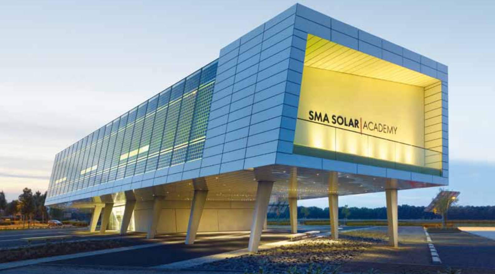
Multicaster-Box 12: SMA Solar Academy is a grid-independent, state-of-art equipped seminar facility built to accommodate 400 people and is located at SMA headquarters in Niestetal, Germany.
