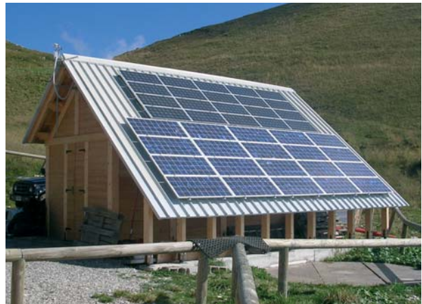
Fig. 9.2: An Alpine hut supplied with PV electricity
