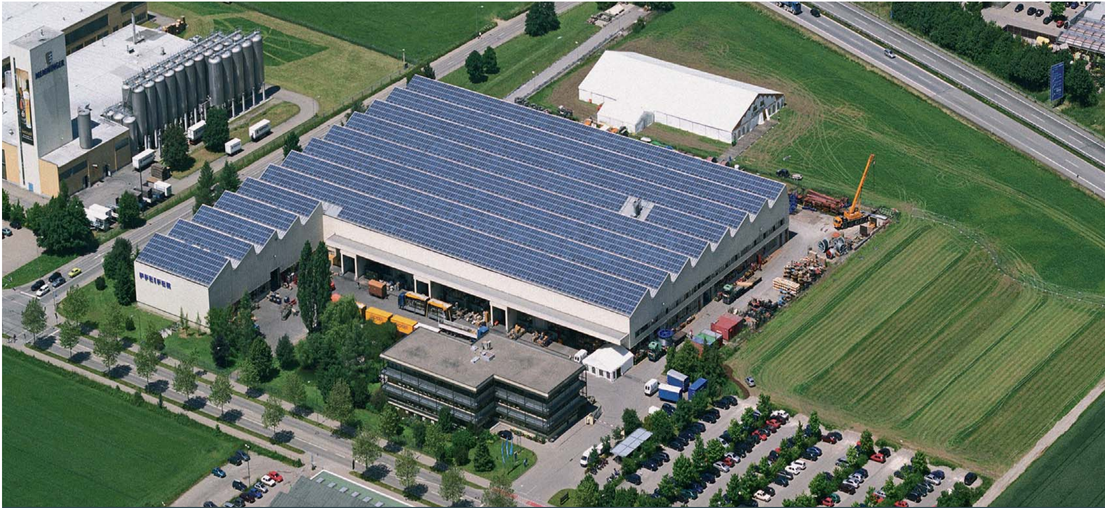
MANUFACTURING BUILDING PFEIFER
